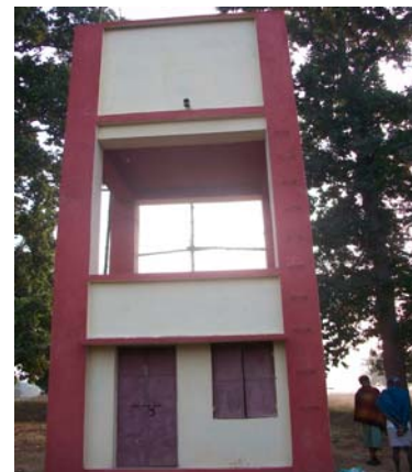
Water Tank for 24 hours water supply
