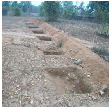
Trenching and Bunding at Sundargarh
