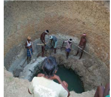
Kathumara well under repair, Damkuda GP in Sundargarh
