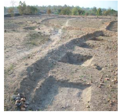
Trenching and Bunding
