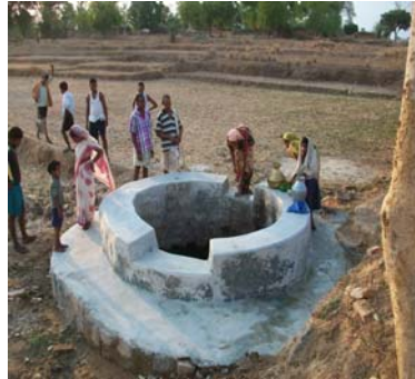
The same well after renovation.
